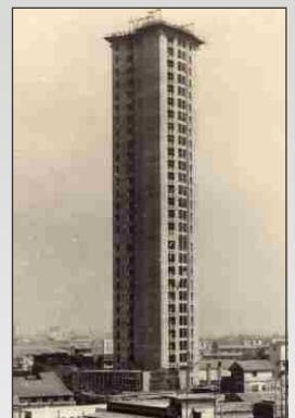
The slip-formed core
