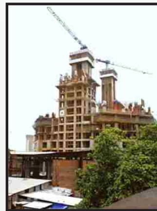
Automatic climbing formwork for cores
