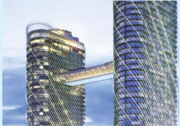
Connecting Bridge between Towers
